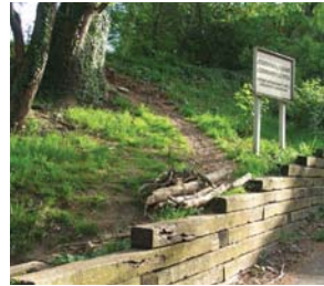
Water moves down from a surface parking lot along a pathway. Retaining wall to slow erosion.
